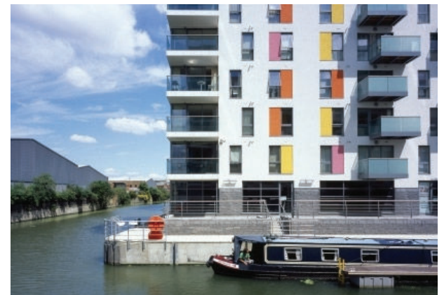
New canal basin, Abbots Wharf, Jestico and Whiles Architects
