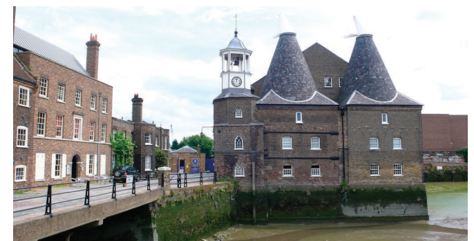
The A12 and railway bridge form the perimeter to the west and south of the site, with the Lea Navigation Canal and Three Mills to the east.
