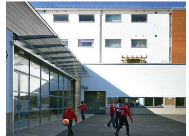
Primary school with housing above, St Jude + St Paul's Primary School, Islington, PTE Architects
