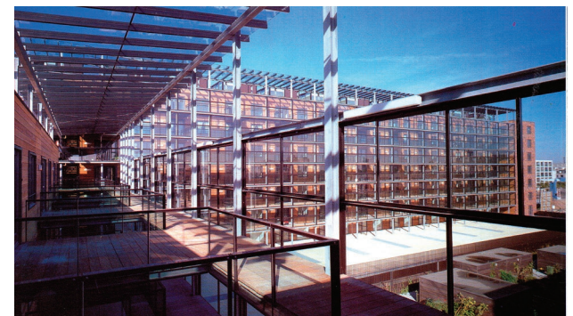
The use of separated access decks could provide an environmental buffer and animated frontage for housing facing the A12. Kop Van Zuid Housing, Rotterdam, KCAP Architects
